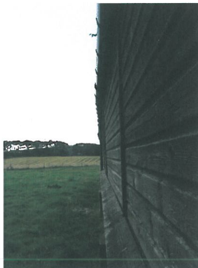
3.4 East Elevation showing signs of bowing in wall.
