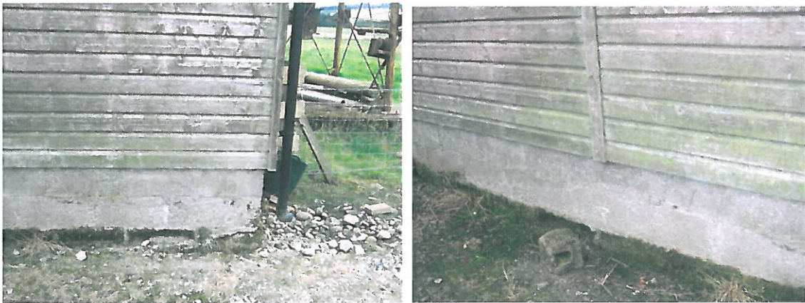
3.7 North Gable wall showing signs of deterioration at ground level.
